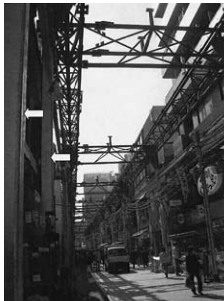
Photo 1 Exterior appearance of an arcade 3) , as an example where JFE Kakuhots are used as columns (white arrow)
