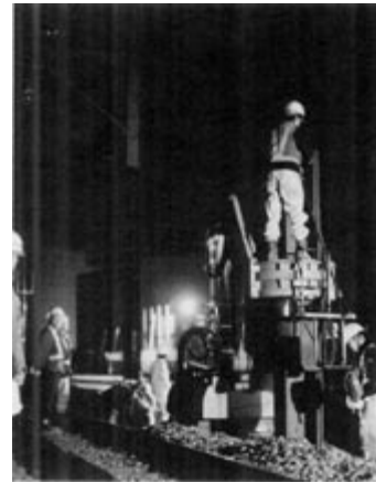
Photo 2 H-shaped steel sheet pile(K-Domeru)
