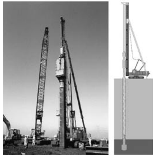
Photo 8 Inner pile excavation method of steel pipe (KING method)
