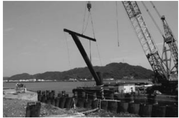
Photo 4 Strutted frame quay-wall structure
